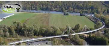
Curvoduc<sup>™</sup> can also achieve very tight bends, such as this conveyor which supplies a thermal power plant with coal at 600 t/hr from the barges from the Moselle river. Thanks to the 250 and 300 m radius bends, the S shape means that a single conveyor belt can be laid down instead of 3 straight conveyors. Fitted with 1,200 mm of belt, this Curvoduc<sup>™</sup>, over 1km long, crosses a canal and ash yard.
